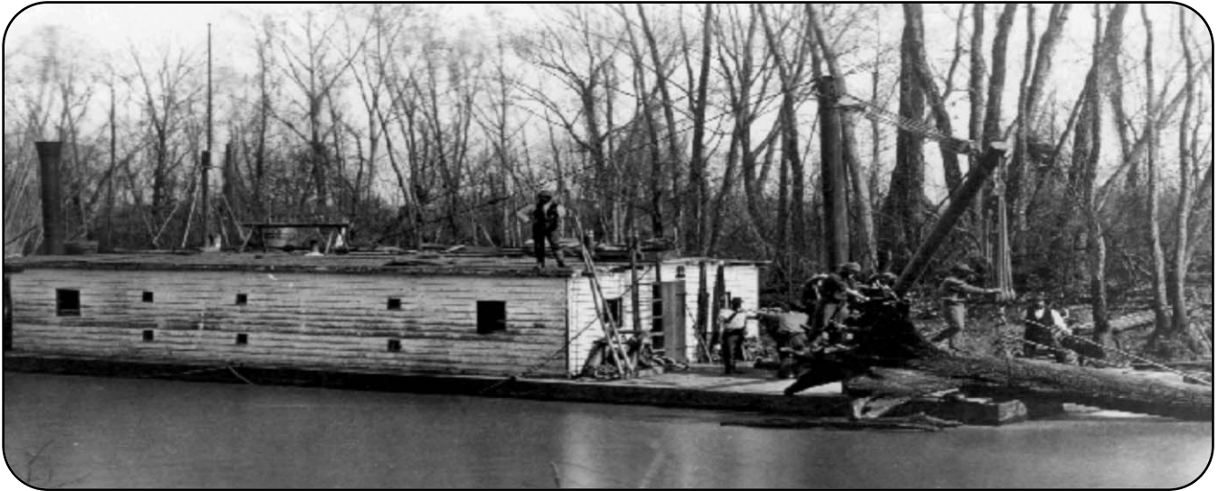
Historic photograph of the Red River raft being cleared courtesy of U.S. Army Corps of Engineers (circa 1873).
