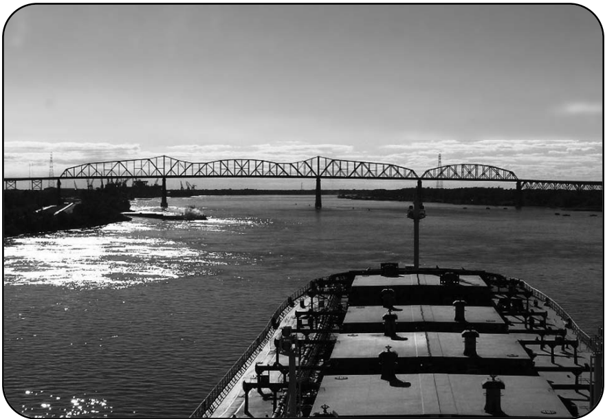
Photograph of barge approaching Huey P. Long Bridge courtesy of New Orleans Baton Rouge Steamship Pilot Examiners.
