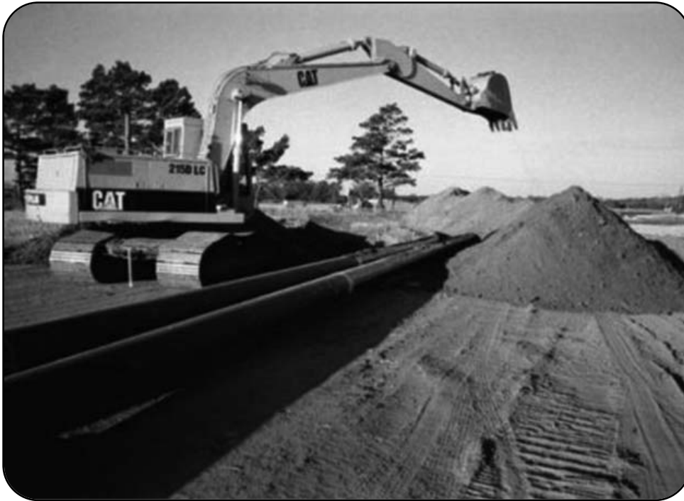
Photograph of gas pipeline being buried courtesy of the Federal Energy Regulation Commission.
