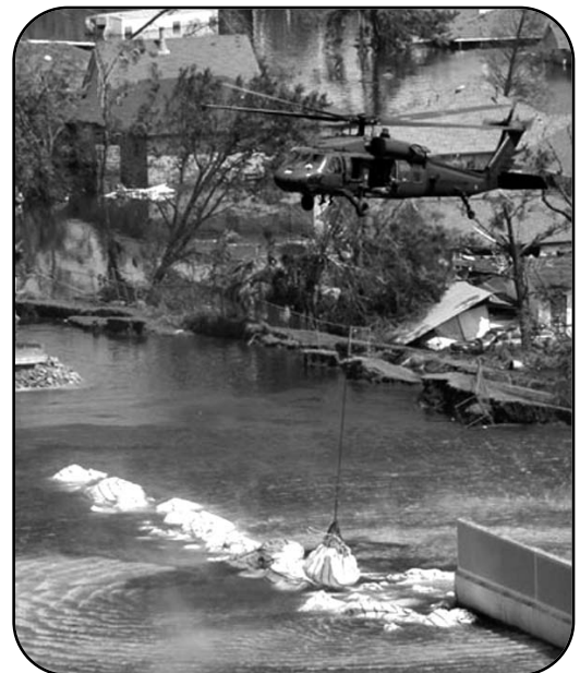
Photograph of levee being sandbagged courtesy of USACE.
