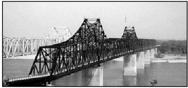
Photograph of Yazoo River Bridge courtesy of the USGS.
