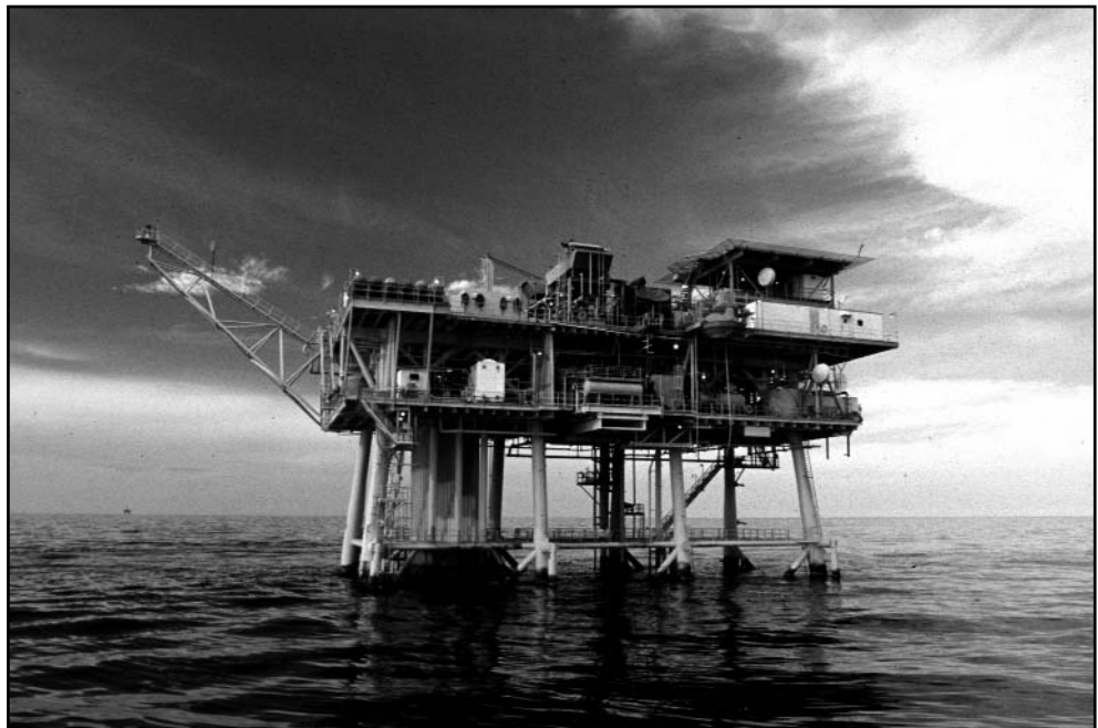
Photograph of oil platform in the Gulf of Mexico courtesy of ©Wolcott Henry 2005/Marine Photobank.
