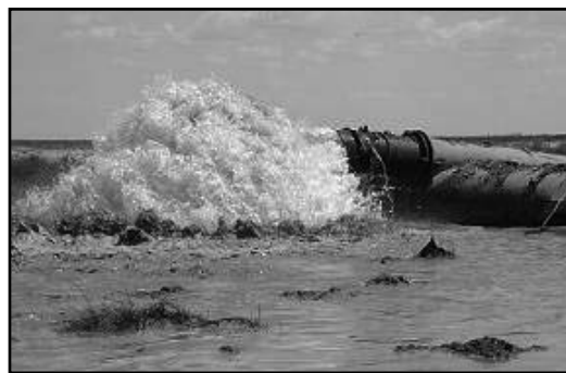
Photograph of pipeline depositing sediment courtesy of the Coastal Protection and Restoration Authority of Louisiana.
