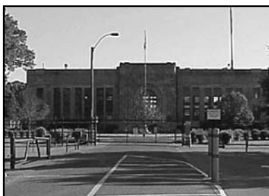
Photograph of Sheahan Pumping Station courtesy of Memphis Light, Gas, and Water Division.
