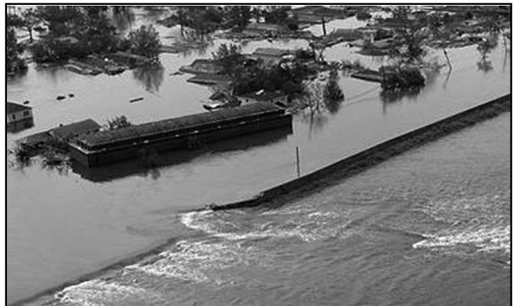
Photograph of New Orleans levee break courtesy of FEMA.
