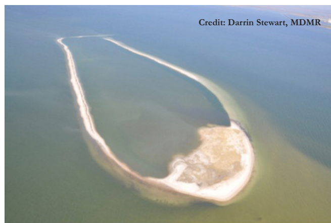
Figure 1. Round Island 2013 - Phase #1 – Looking northwest (training dike and initial island habitat)
