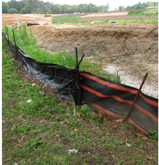
Silt fence used at a construction site in Oxford, MS.
